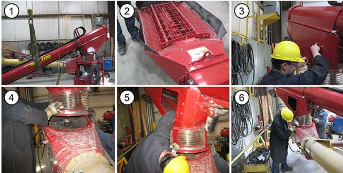
Figure 4. MKX-Tend Hopper General Installation
